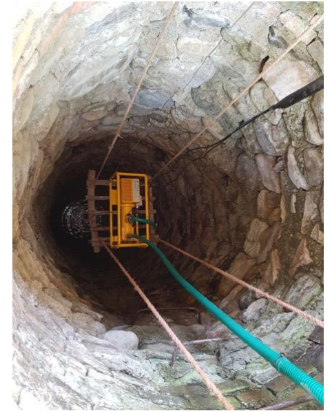
Lower the pump down into the well and closer to the water table if it is lower than 7 meters
